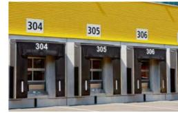
Continuous vertical/horizontal rooflight, sectional gate und loading technology
