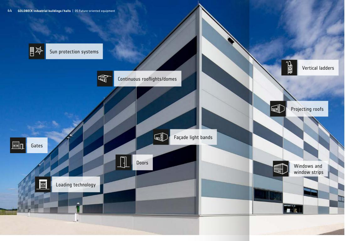
Vertical light bands, continuous rooflights/domes and projecting roof
