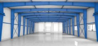
Frame structures: truss beam and crane track (top) and with solid wall profiles (bottom)
